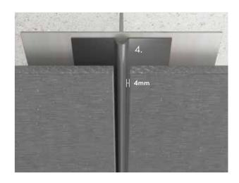
Cembrit Caulking Profile can be used in both vertical and horizontal joints. It is not mandatory to use Cembrit Caulking Profile, but it provides excellent joint solutions. The profile is installed in the same way as Cembrit External Corner.
