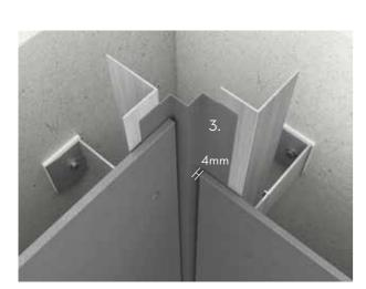
Cembrit Internal Corner is used for 90° internal corners. Secure the profiles with double sided tape. Once fixed, the facade board will secure the profiles in position. There should be a minimum 4mm gap between the board edge and the profile.
