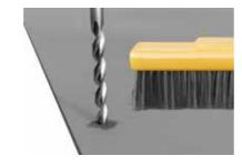
If not using Cembrit Facade Wing Screws, the boards should be pre-drilled with an appropriate fibre cement drill bit. Dust from cutting or drilling must be removed with a brush immediately after the work has been completed, otherwise it can mark the surface of the boards.
