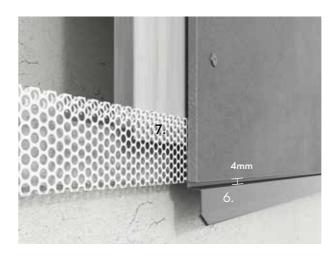
Cembrit Drip Small is used to drain water away from the supporting structure or where neat detailing is required at the foot of the facade. The profile can be used in conjunction with Cembrit Ventilated Profile to ensure that insects and vermin cannot enter the cavity behind the facade boards. There should be a minimum 4mm gap between the board edge and the profile.
