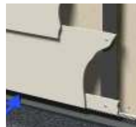
Start with a small strip of panel at the base.
